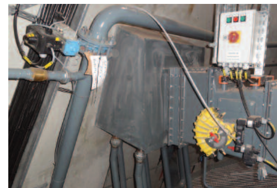
6. Silo mounting frame for discharge of inner silo
