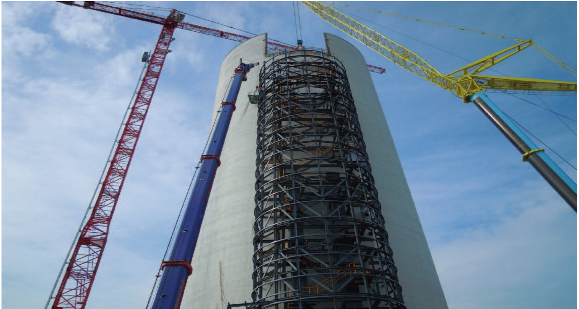
6. Erection of staircase tower
