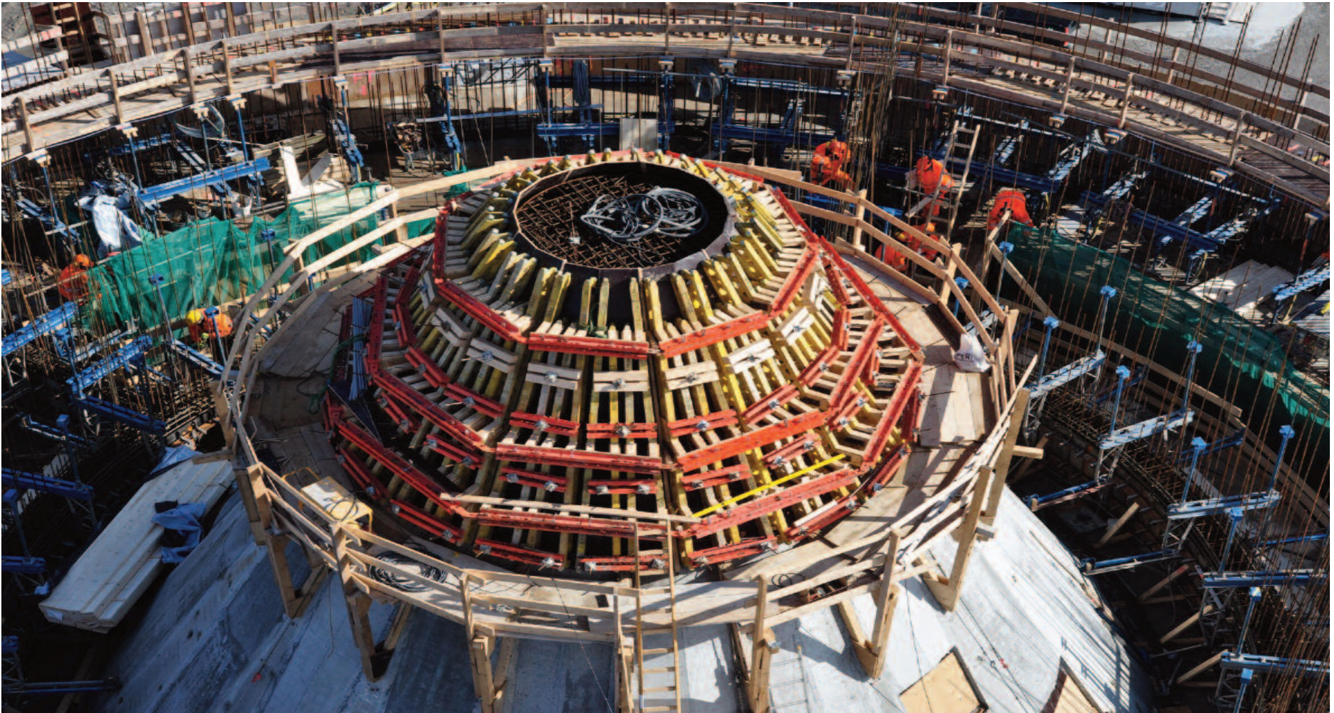
2. Casting of upper cone
