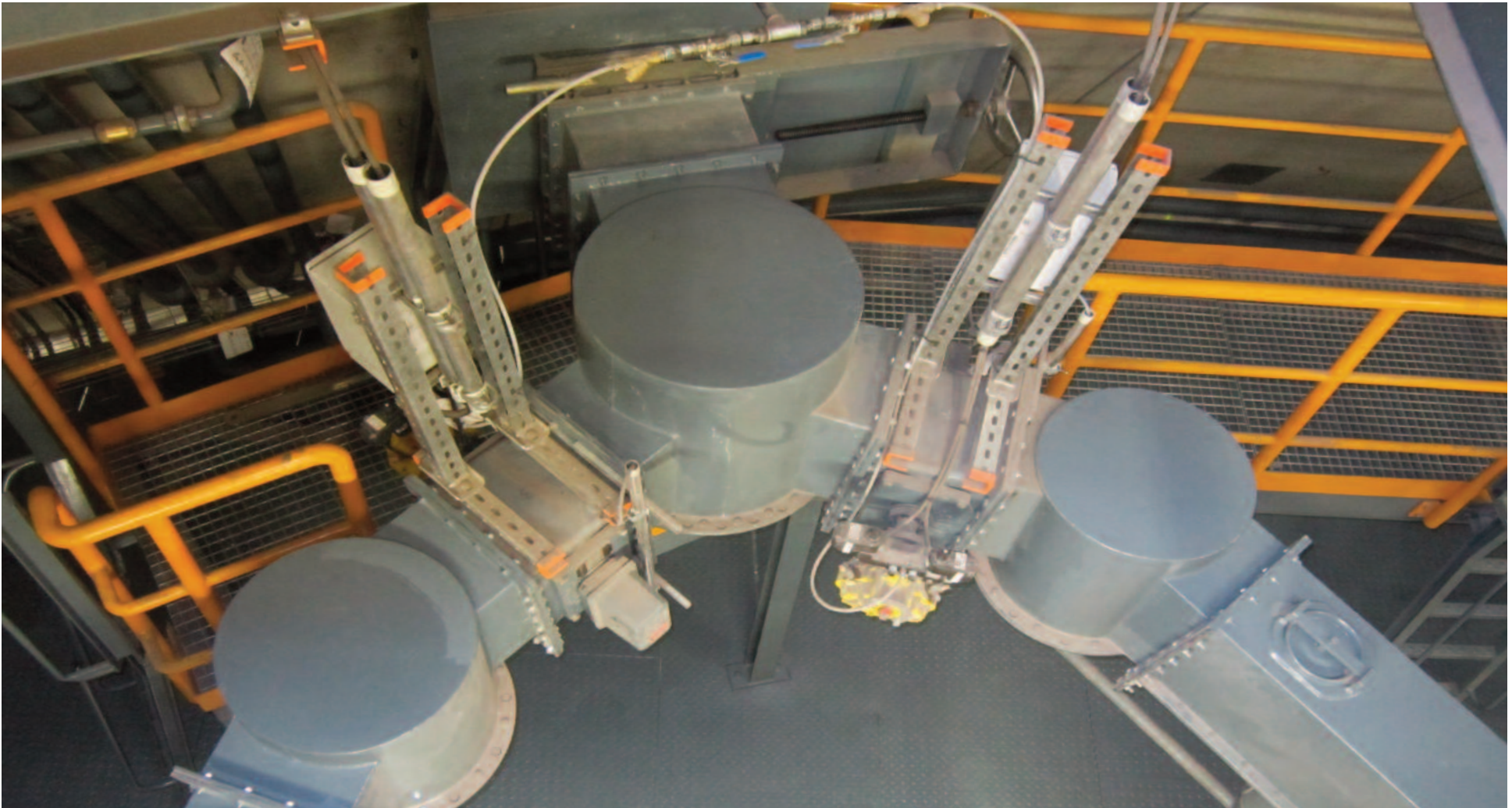
3. Typical silo discharge section
