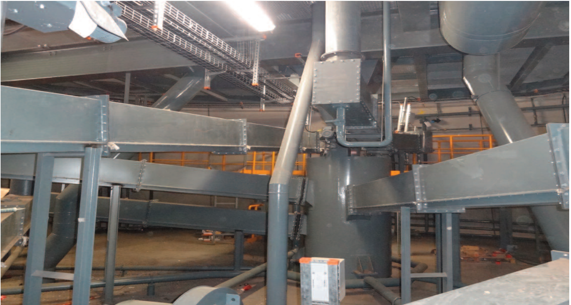
1. Transport for silo discharge airslide
