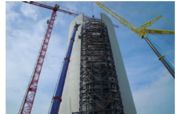
6. Erection of staircase tower
