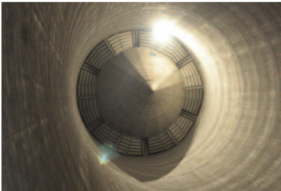
4. Top view of central chamber with 10.000 t capacity
