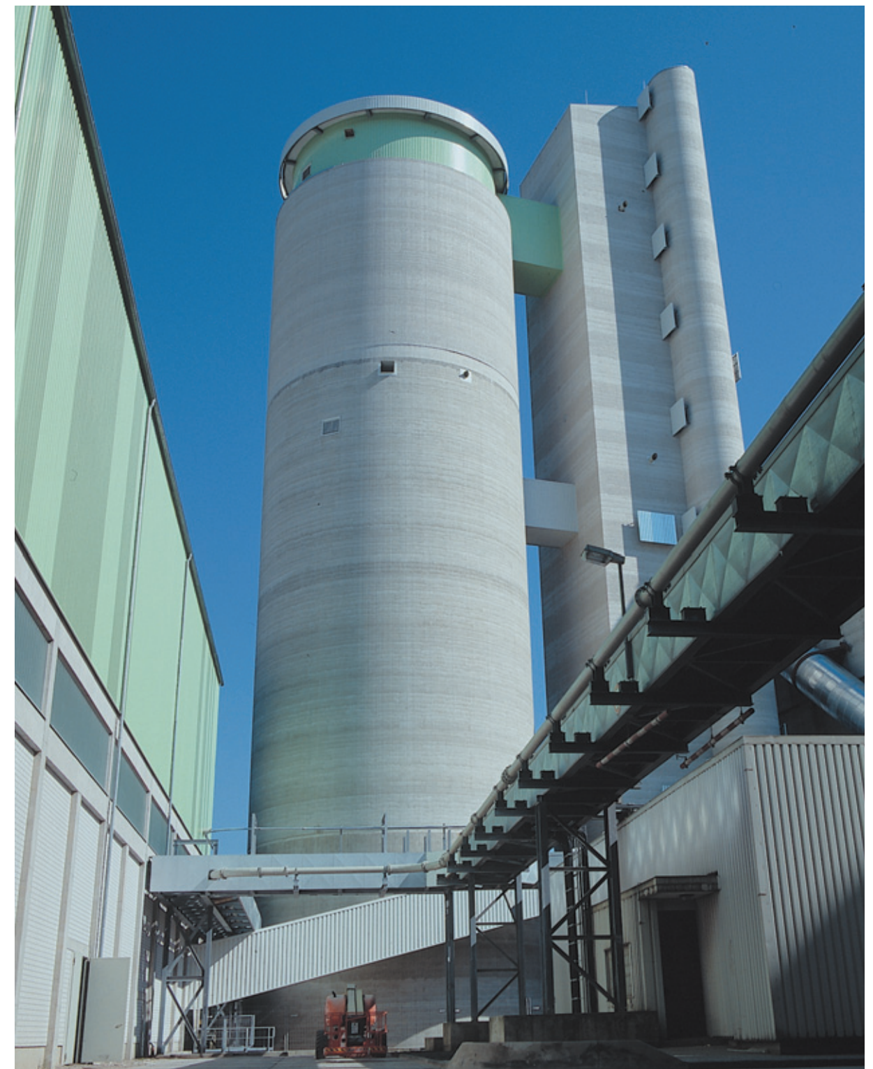
Raw meal silo for Dyckerhoff Cement works, Lengerich, Germany
