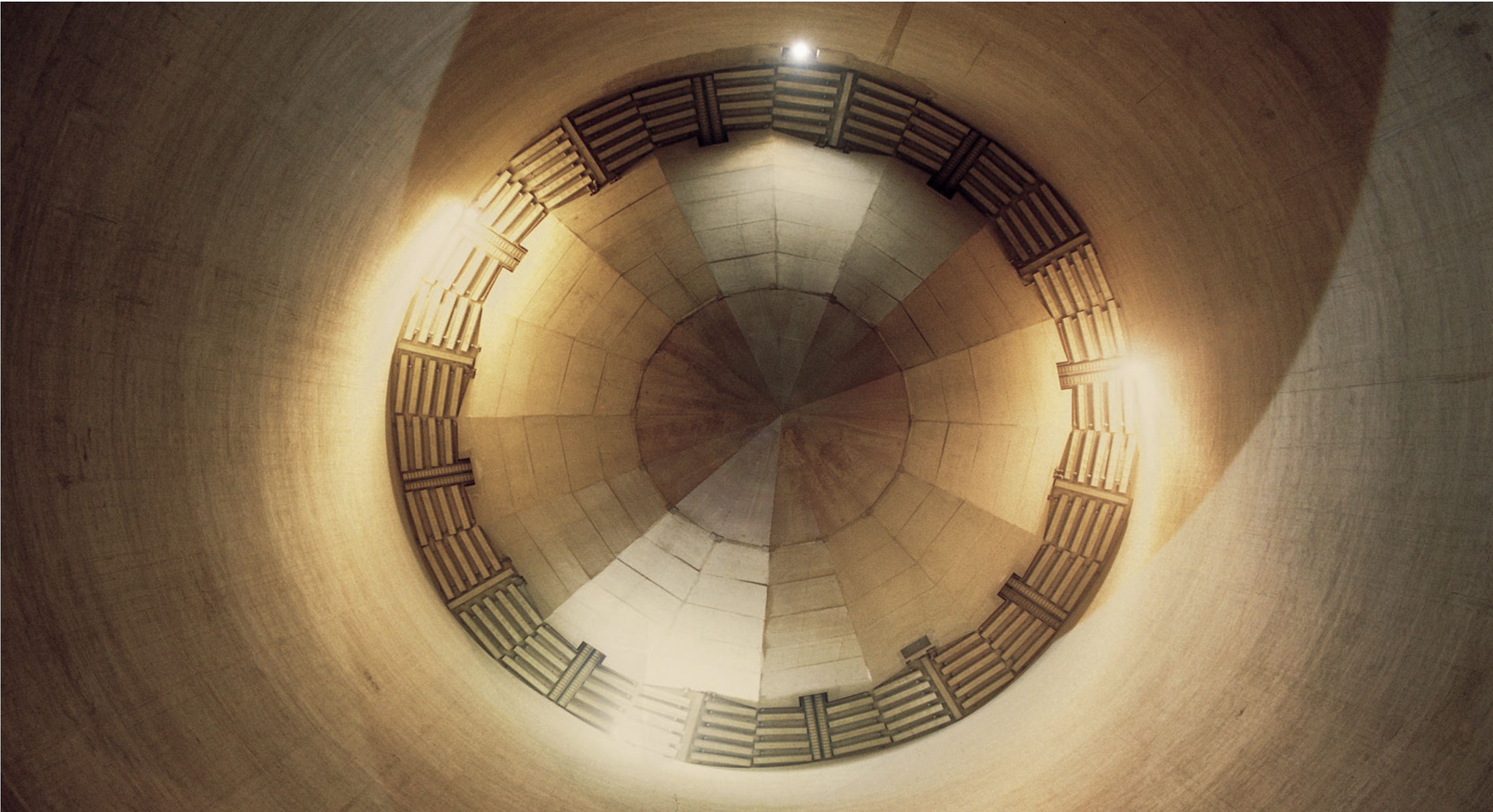
View into the central cone silo with ring shaped bottom and fluidslide system
