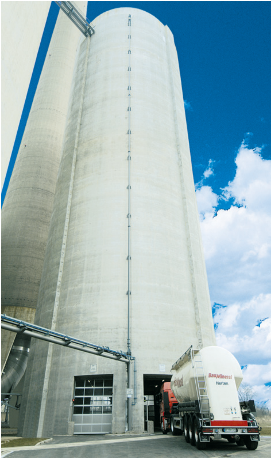
The IBAU Central cone silo 25.000 m³ at the Mehrum Power Plant
