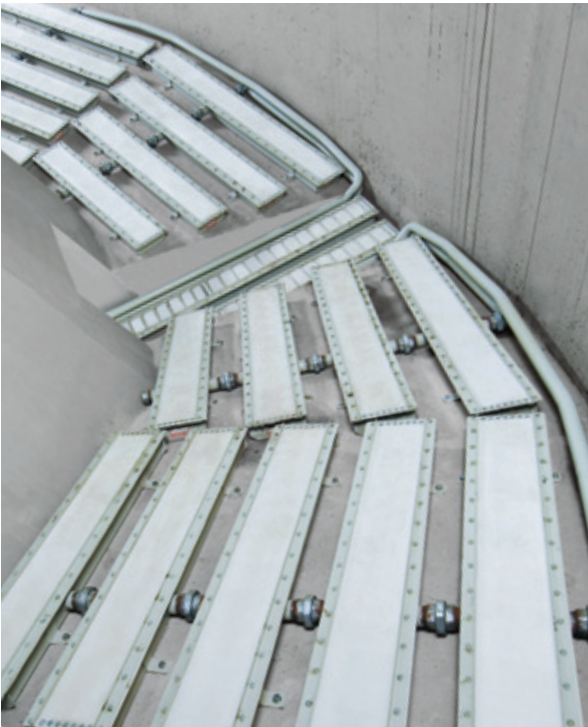
Aeration section and silo outlet
