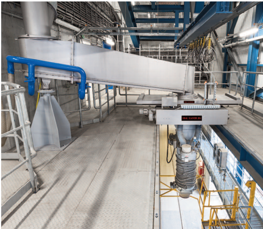
Mobile truck loading system for dry fly ash
