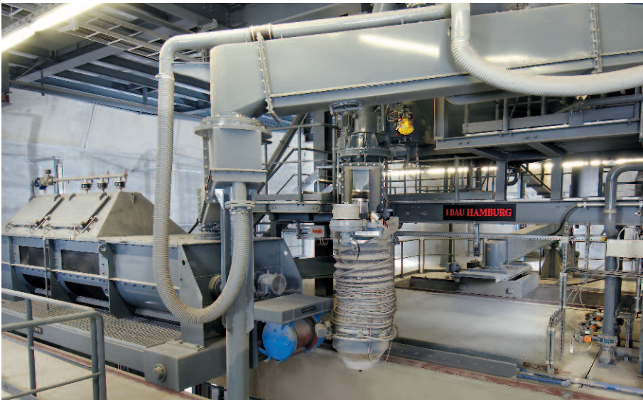
Combined dry ash and movable wet ash loading system
