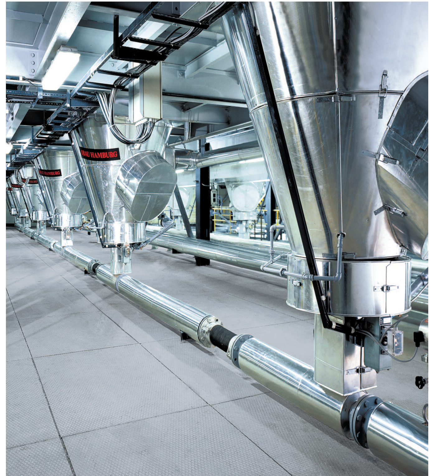
Pneumatic conveying of FGD-Product by pressure vessels
