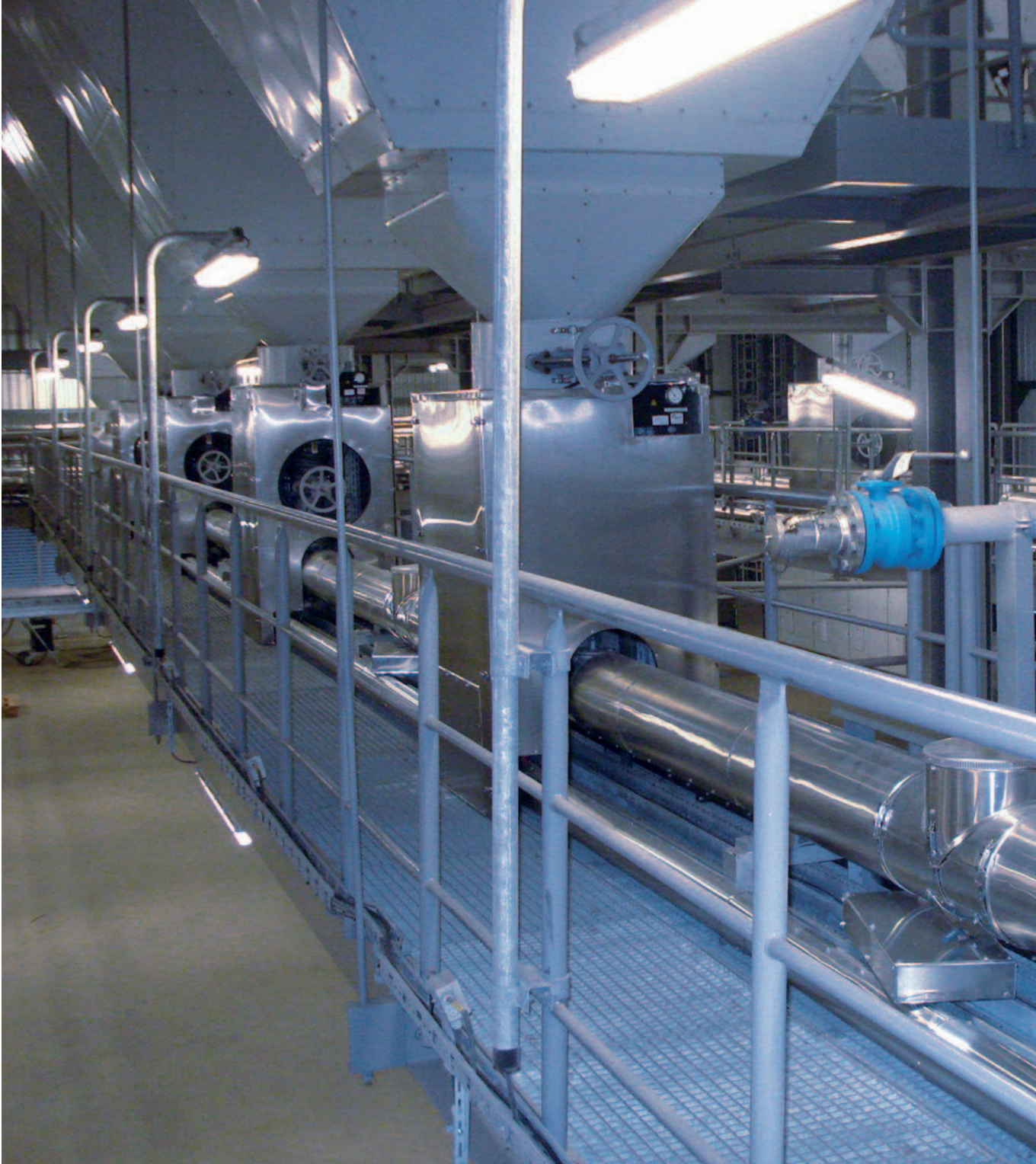
IBAU Fpipe for a fly ash removal system of an ESP
