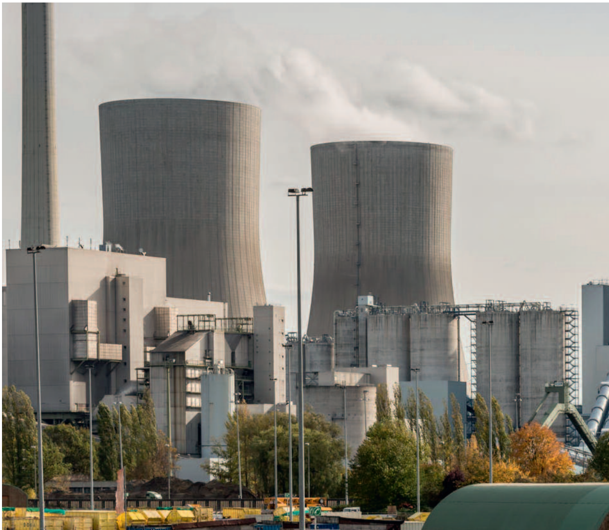
Limestone and fly ash storage silos for RWE STKW Westfalen, Germany
