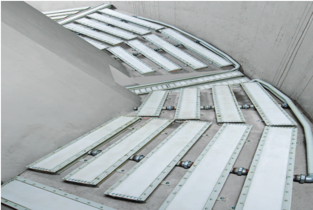
Typical discharge section of an IBAU Silo
