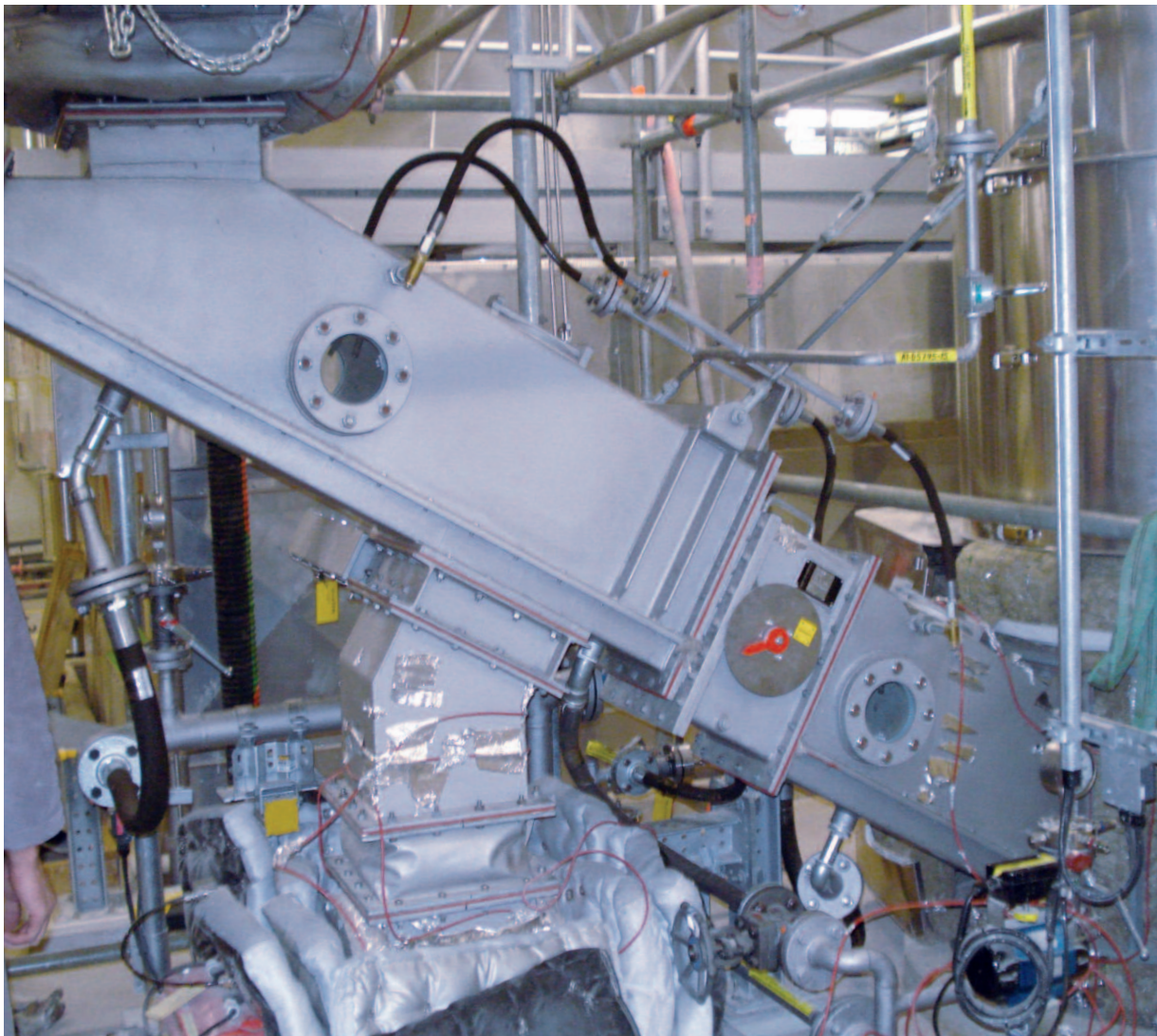
Feeding system of hydrated lime into the flue gas scrubber
