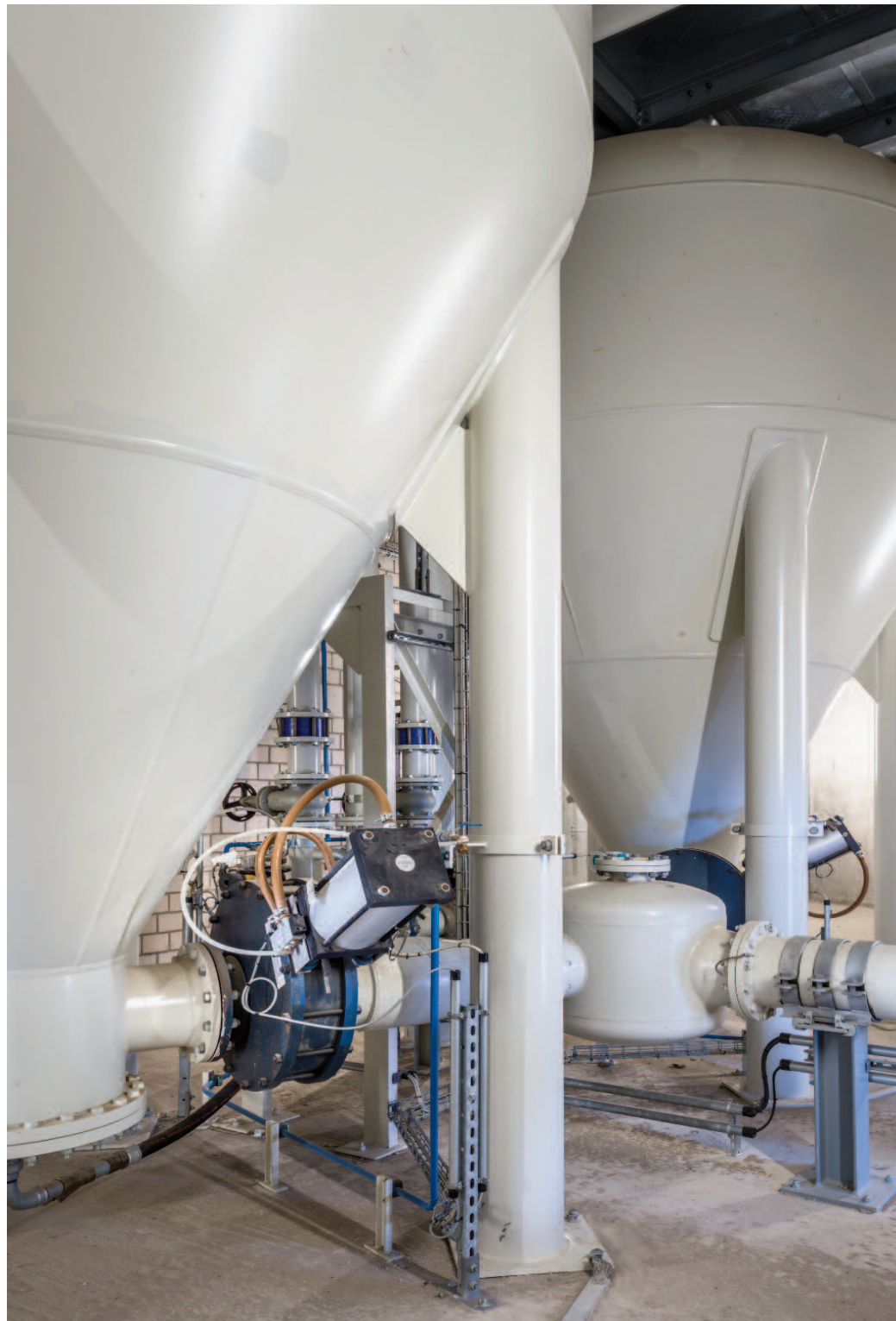
Pneumatic fly ash conveying system with IBAU Pressure vessels
