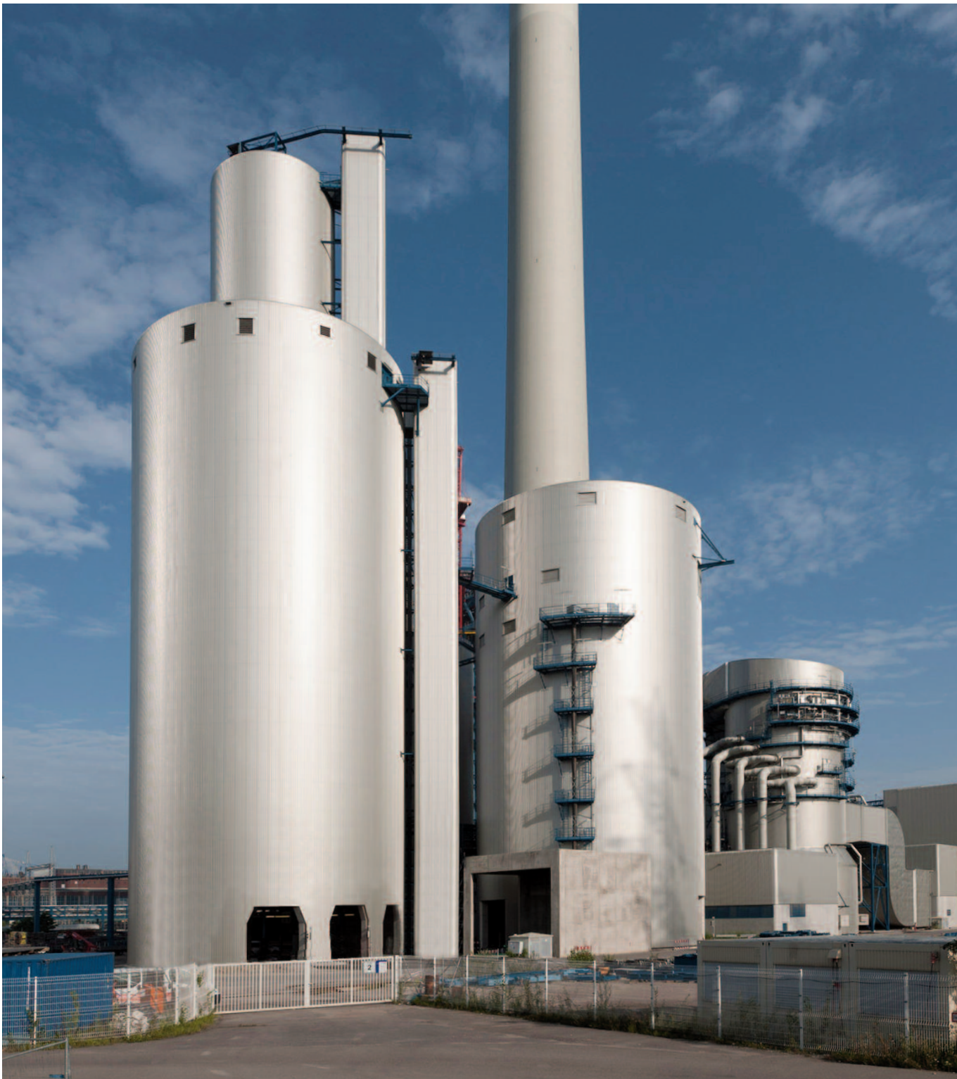
IBAU Fly ash storage silo in a coal-fired power plant
