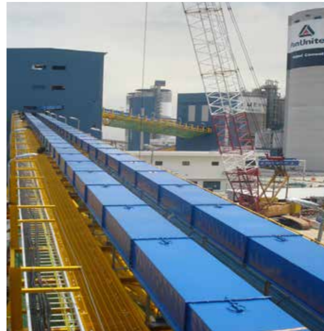
Material handling via airslides
