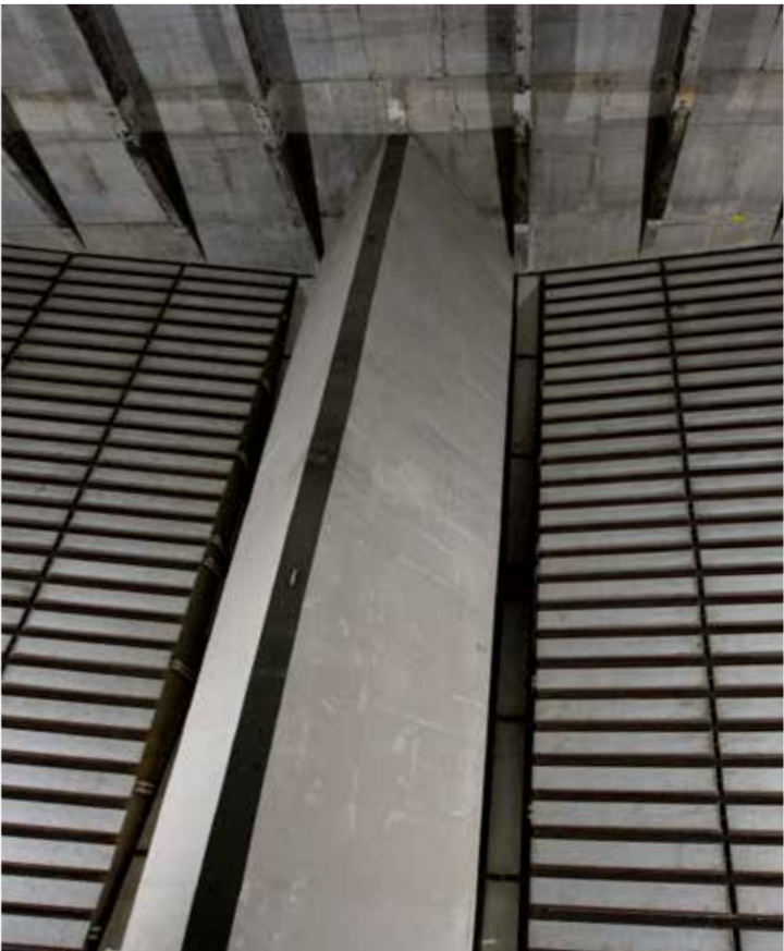
Compartment with fluidslides installed on the bottom
