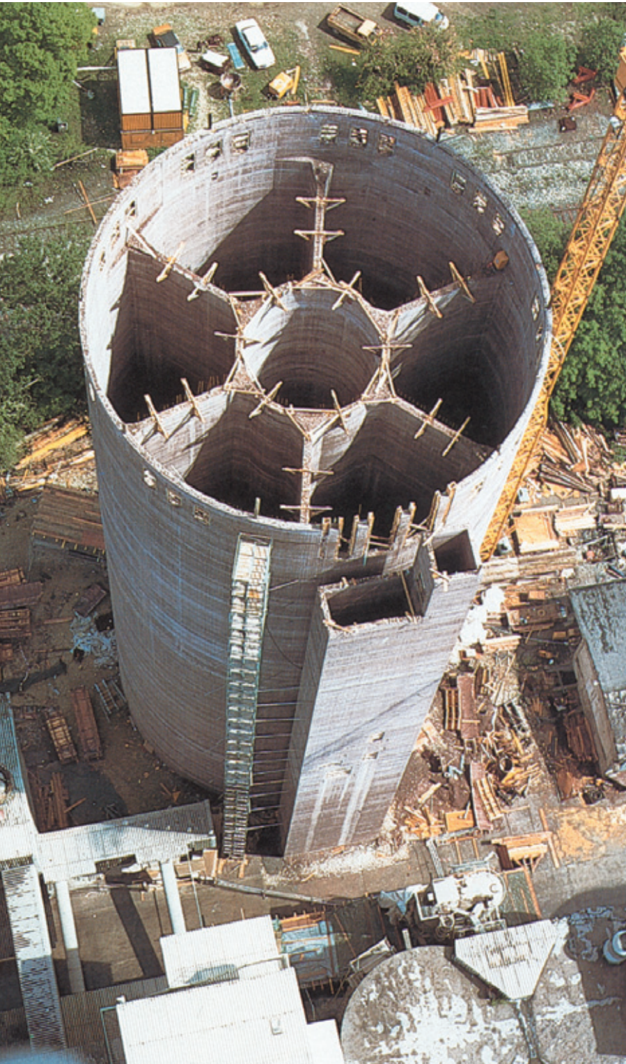
Multi-compartment ring silo during construction
