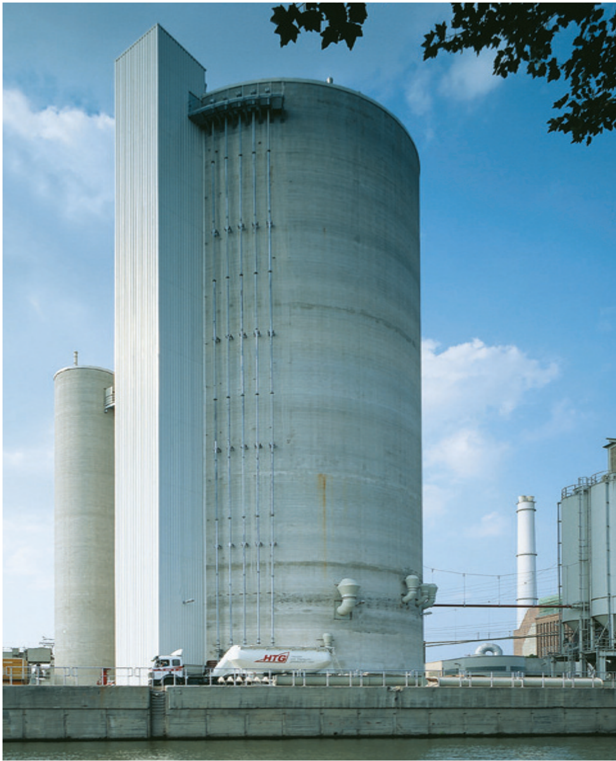
Multi-compartment silo with 11 compartments, silo diameter 24,0 m for Zementwerke Berlin, Berlin, Germany
