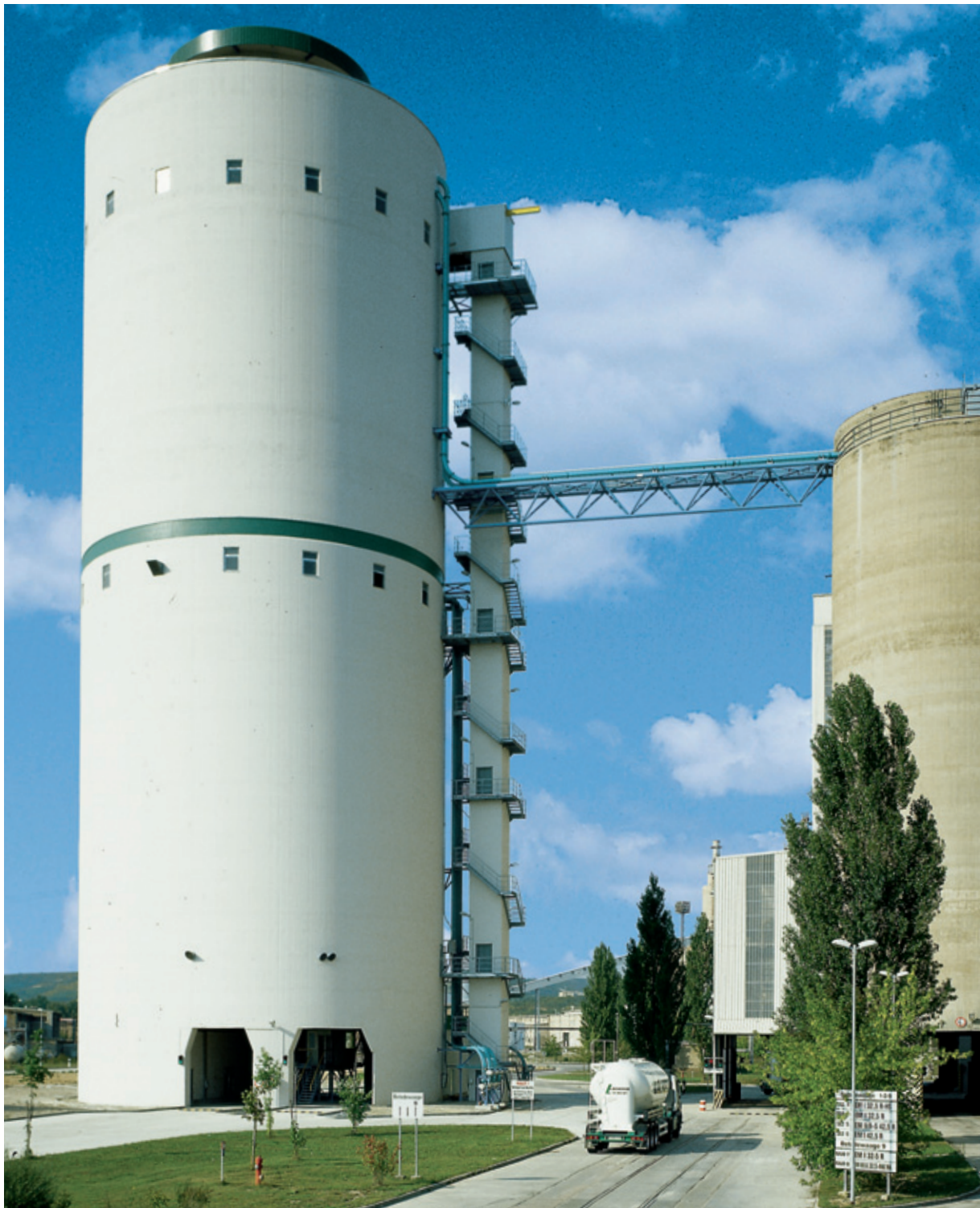
Multi-compartment silo with 13 compartments, silo diameter 24,0 m for Lafarge Zement, Karsdorf Works, Germany
