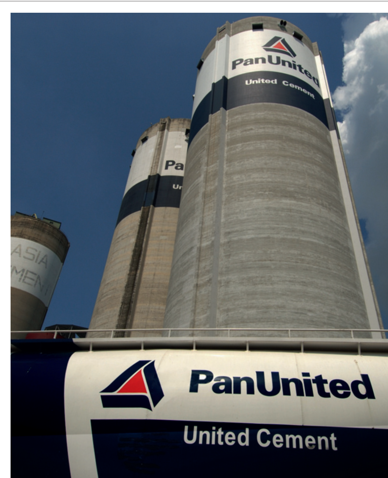
2 Multi-compartment ring silos with 2 compartments each, silo diameter 26,3 m and 24,2 m for Pan United, Singapore
