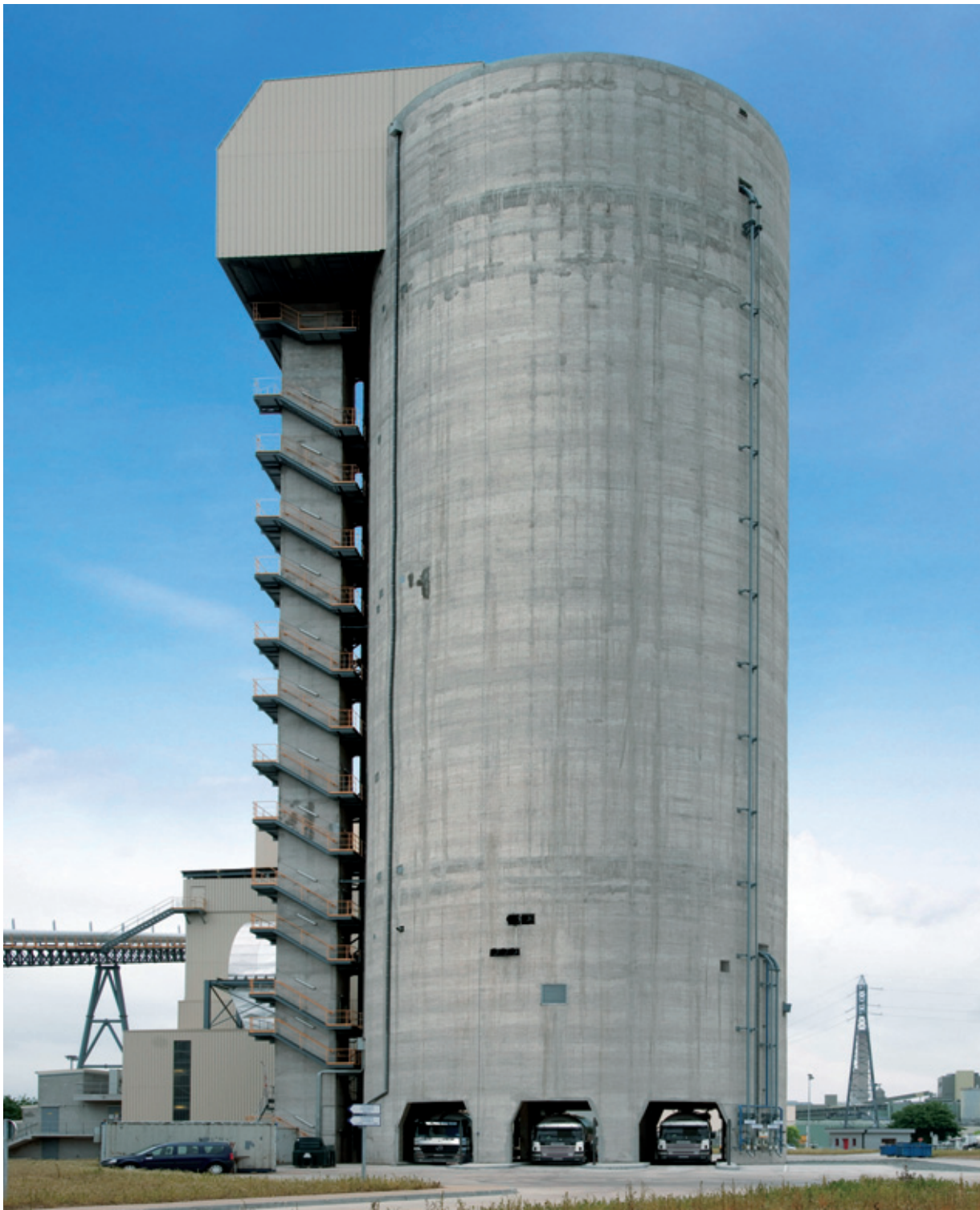
Multi-compartment silo with 7 compartments, silo diameter 21,0 m for Holcim France, Val de Seine Works, France
