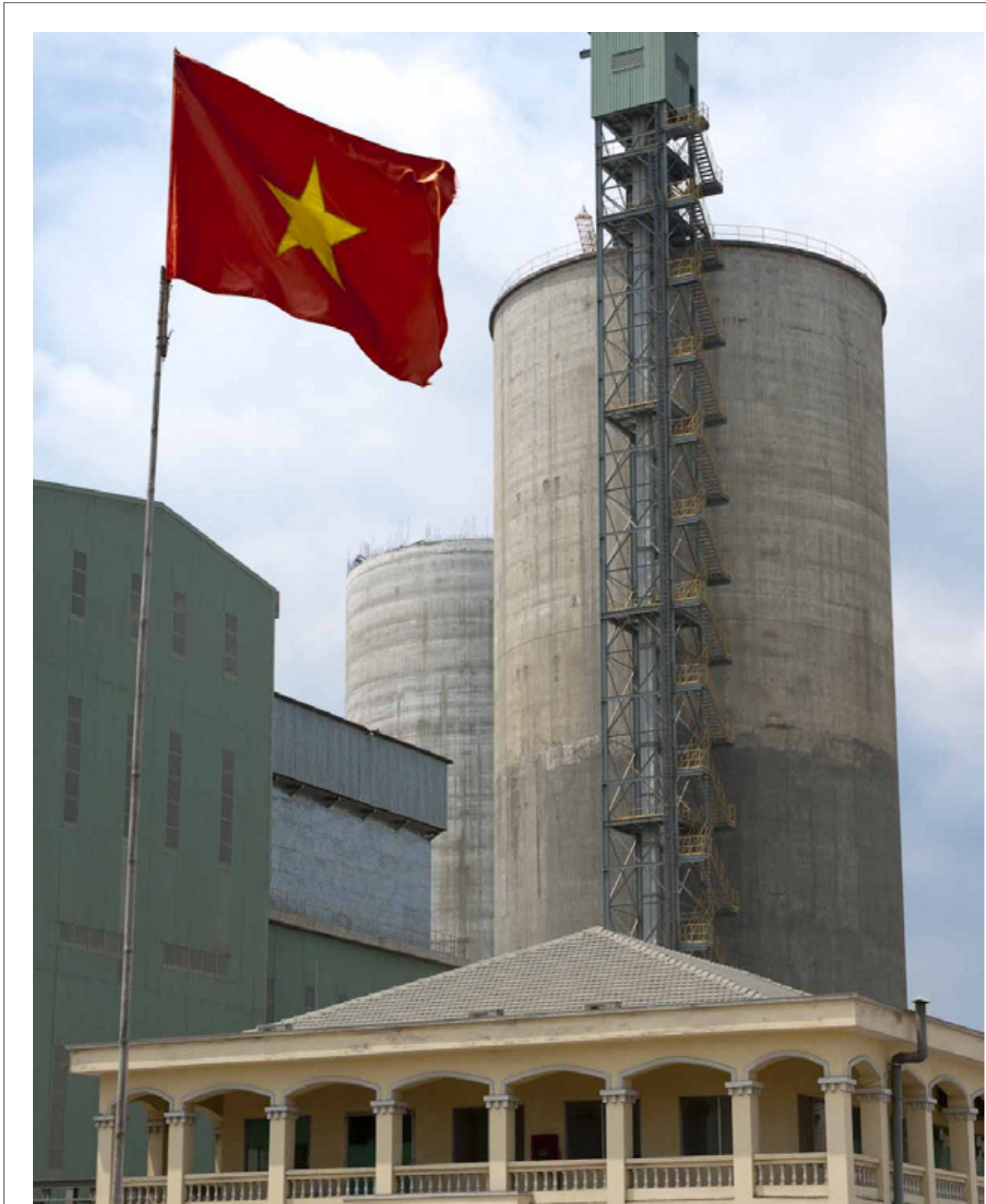
Multi-compartment silo with 5 compartments, silo diameter 28,0 m for Hatien I Cement Company, Ho Chi Minh City, Vietnam
