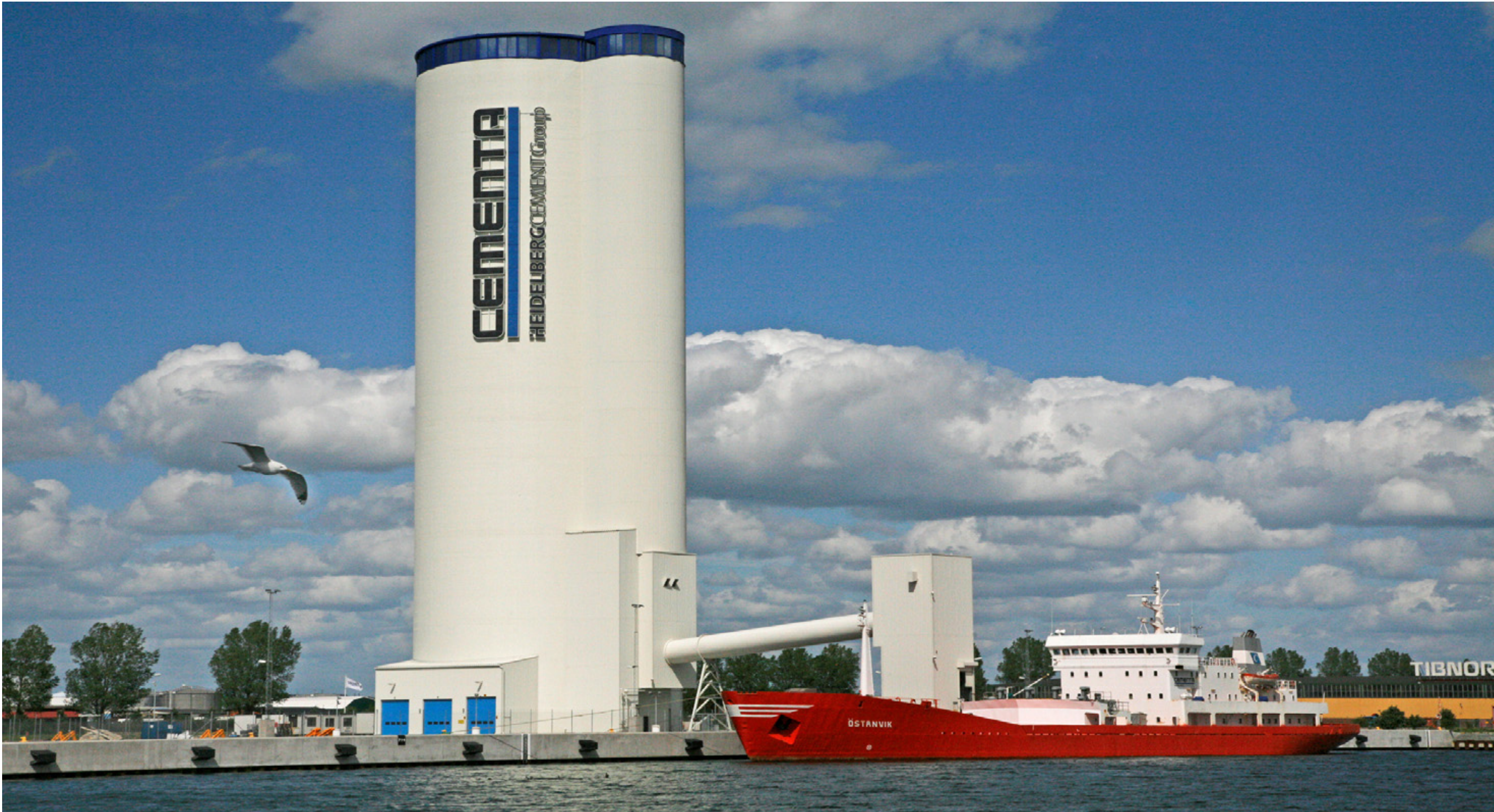
Multi-compartment silo with 6 compartments, silo diameter 26,0 m for CEMENTA AB HeidelbergCement Group, Malmö Sweden
