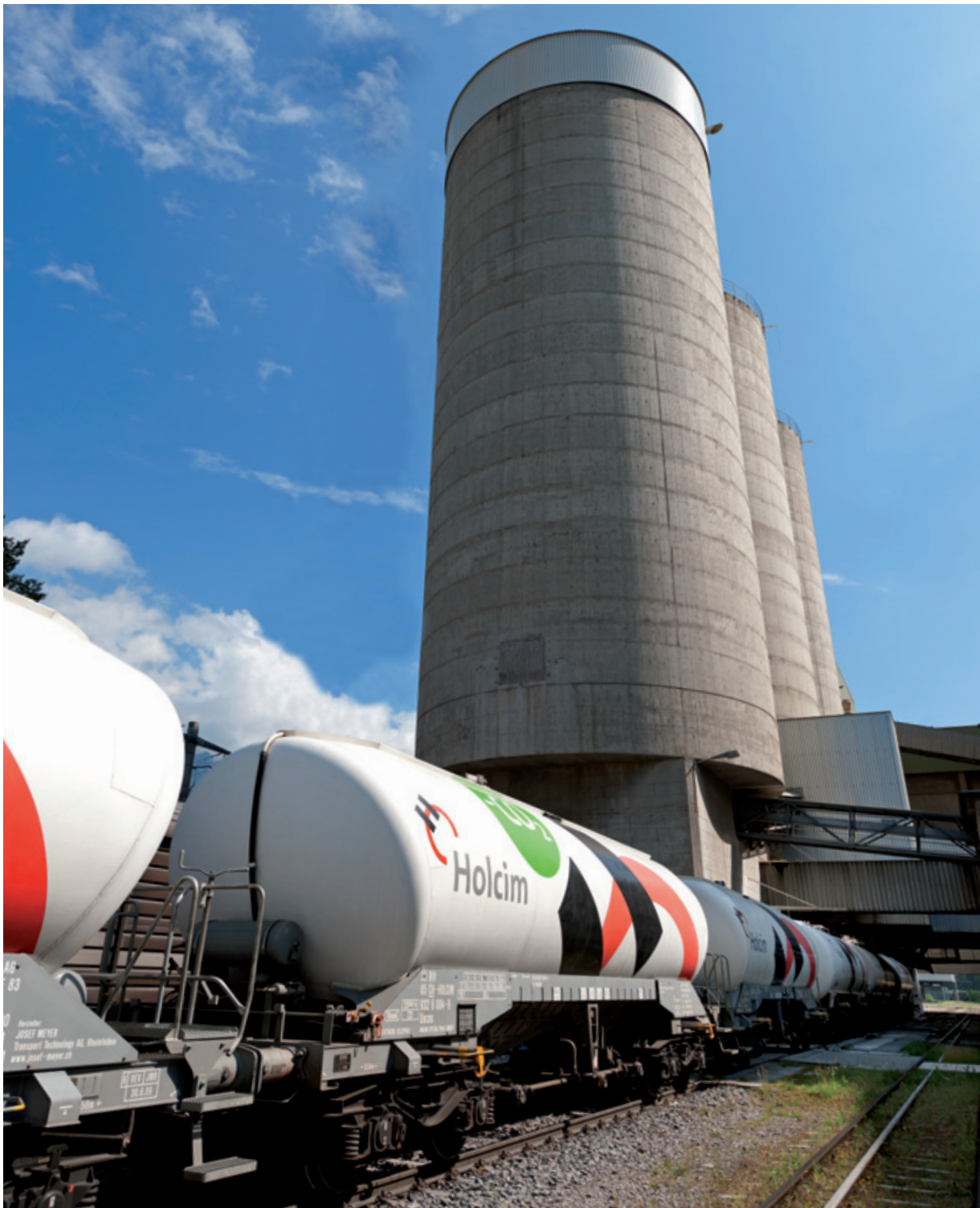
Silo conversion into a multi-compartment silo with 5 compartments, silo diameter 16,0 m for Holcim, Untervaz, Switzerland
