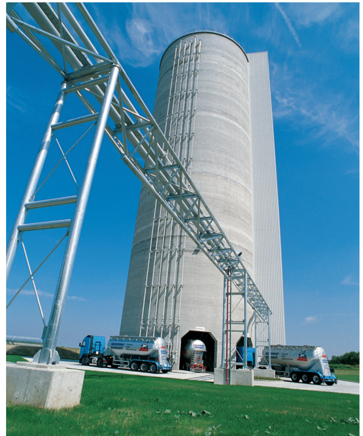
SPENNER ZEMENT Multi-compartment silo with 15 compartments, silo diameter 20,0 m for Spenner Zement, Erwitte Works, Germany
