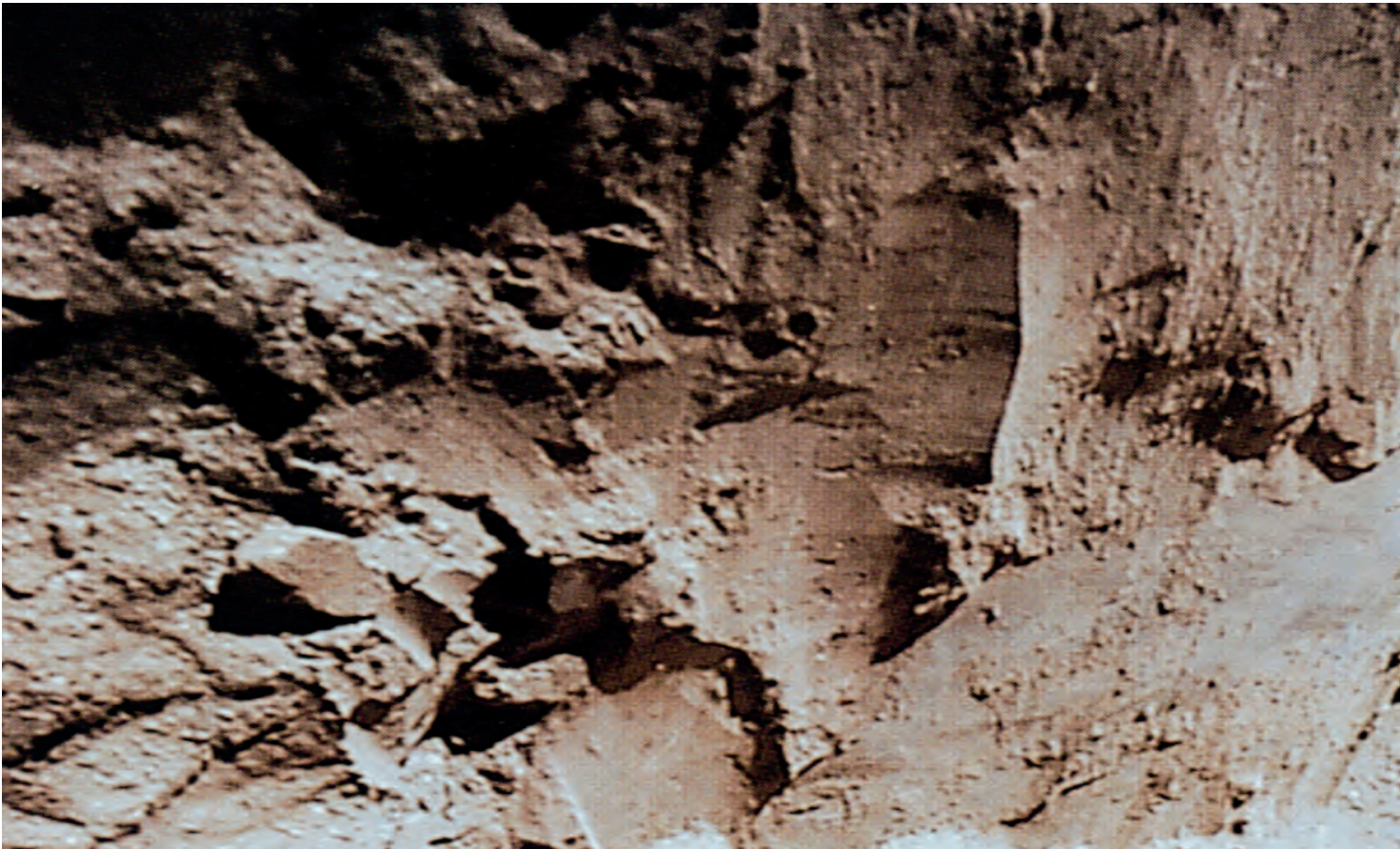
The lumps shown on the silo wall can cause problems at the silo discharge
