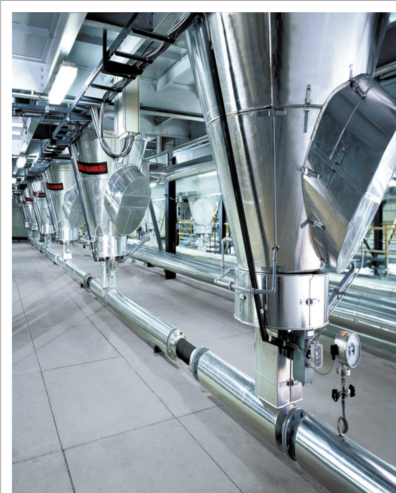
IBAU Pressure vessels in the Litvinov power plant
