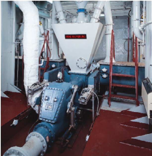
Cargo holds with aeration panels and fluidisation system with feeding of the IBAU Pump
