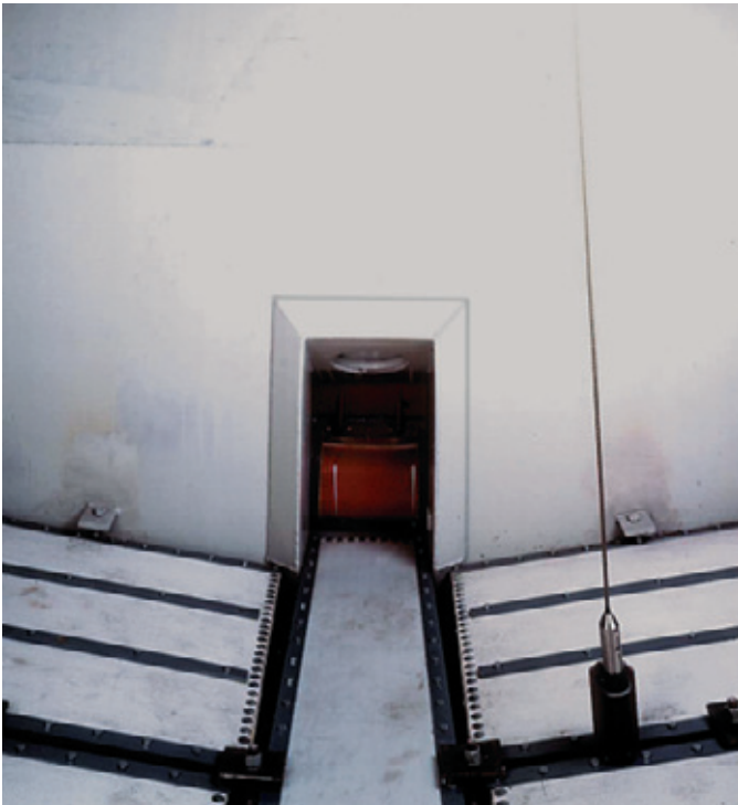
Cargo hold discharge
