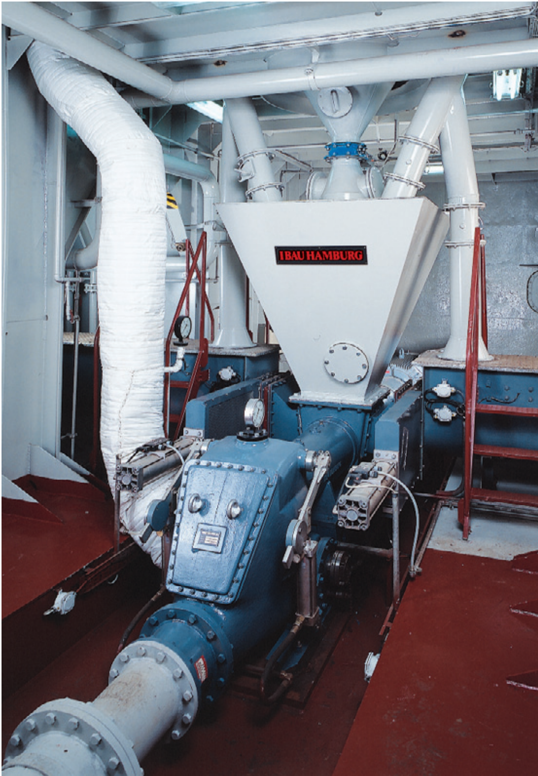
Feeding of IBAU Pump
