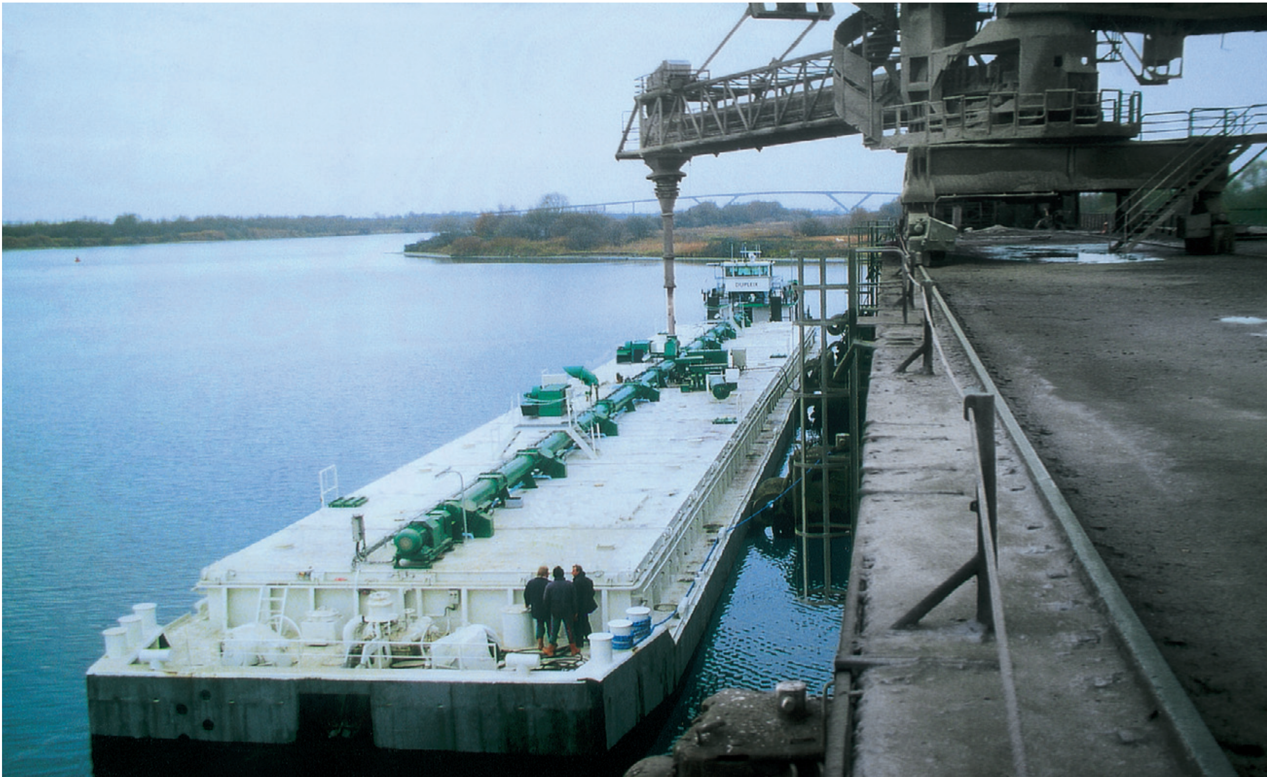
Loading station for LAFARGE CEMENT at Le Havre port
