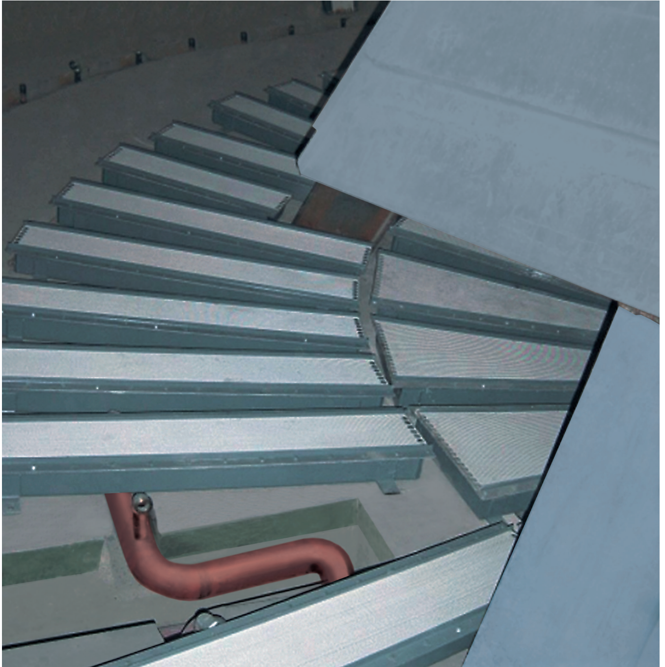
Floor aeration panels outside the steel cone
